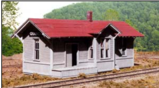
DT&I Standard Station, Waiting Room Right
